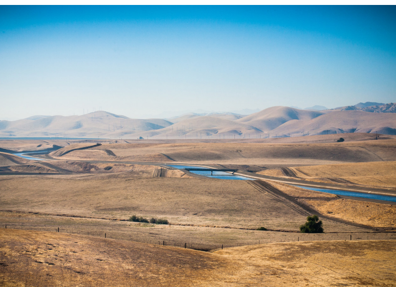
The State Water Project, running through the Central Valley, is the largest state water infrastructure project in the country.
